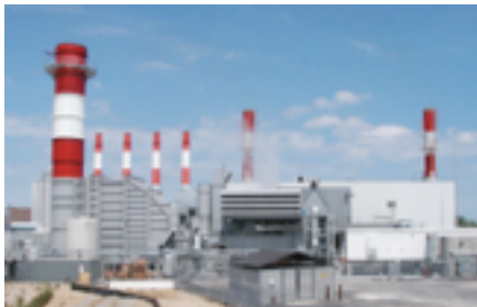
Bethpage 3rd Turbine Peaker Power Plant Project, 50MW, 50 MM 1 year
