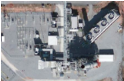
Santa Rosa Energy Centers, 240 MW CHP 155 MM 1yr build time 2 Modular Units
